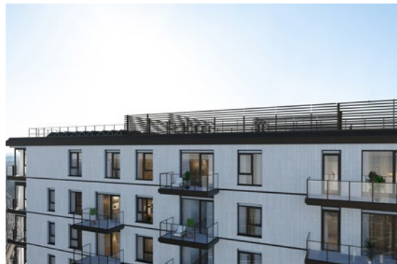
Roof Terrace – View South
