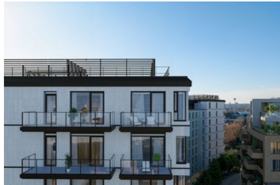
Roof Terrace – View South
